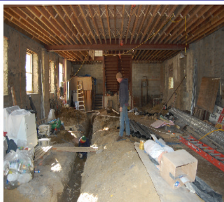
The inside of the building has a loooooong way to go.
